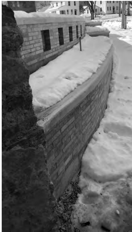
The retaining wall beside the entry plaza.
