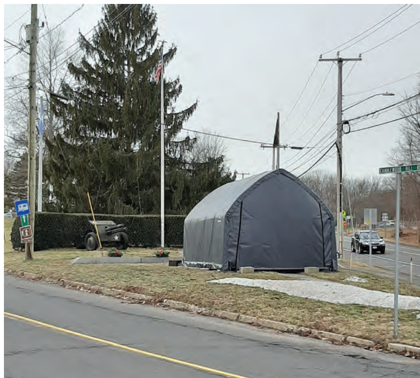
Covered memorial under renovation. Photo by Kim Bodak.
