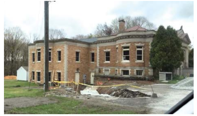
Brainerd Library renovation.
