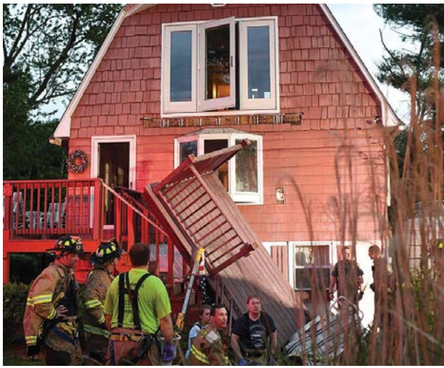
Deck collapse, June 2019. Photos by Olivia Drake.
